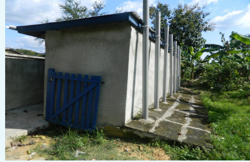
Ventilated pit latrines constructed as part of RI/USAID International Collaboration initiative in Osiem, Ghana. Photo by the Rotary Club of Accra Ring Road Central
