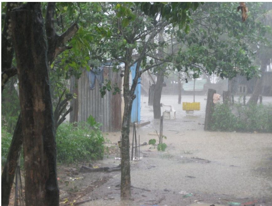
Photo 2: Improperly sited latrine which has flooded.
