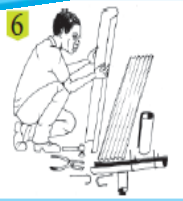
6 Cut out iron sheets to make gutters and delivery pipe. Use wires to mount gutters onto the roof.
